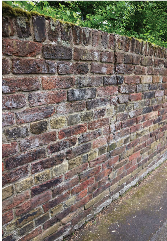
3.2 Evidence of alteration to front garden wall (Insall)
