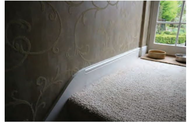
3.15A Mismatched string to principal stair between lower ground & ground floors (Install)
