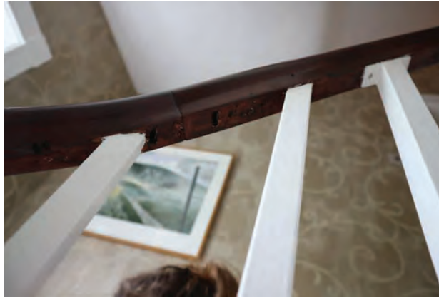
3.14 Alterations to handrail & balusters (Install)
