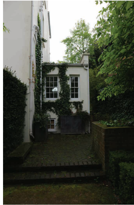
3.10 Rear elevation of entrance wing (Insall)
