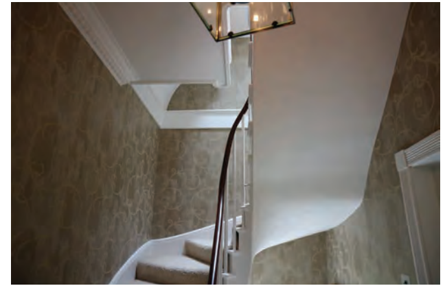
3.16 Original stair profile & underside of later WC insertion (Install)
