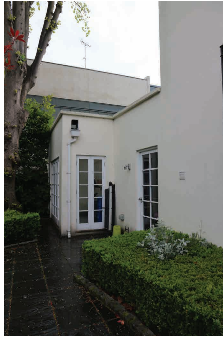
3.9 Rear garden room to modern garage extension (Insall)
