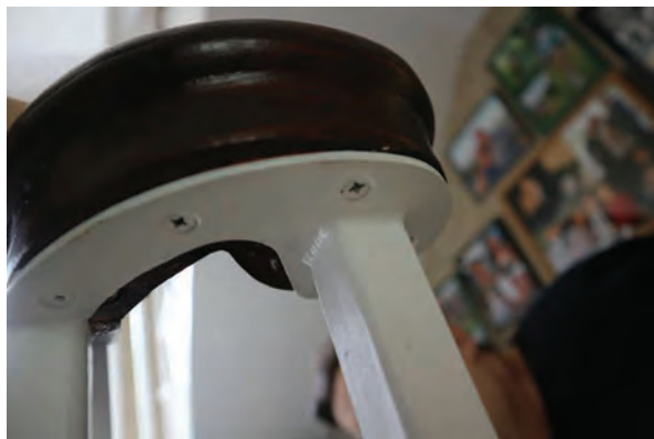
3.12 Lower ground floor newel replacement (Insall)
