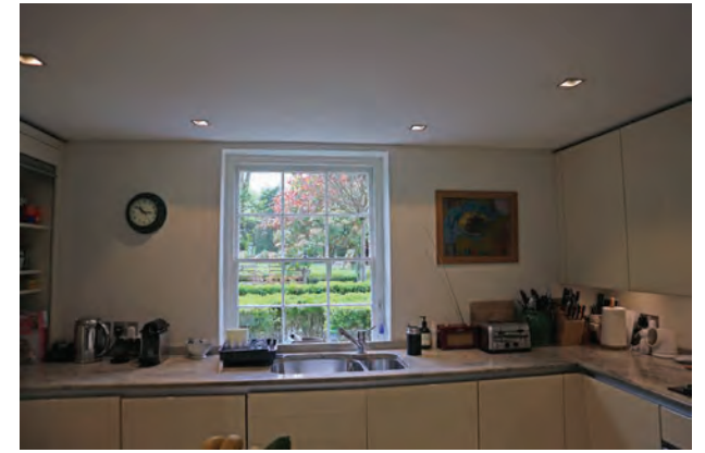
3.21 LG6, truncated window opening (Install).
