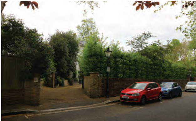
3.3 Western approach to house, shared with no. 12B (Insall)
