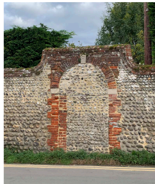
Precedent of brick archway
