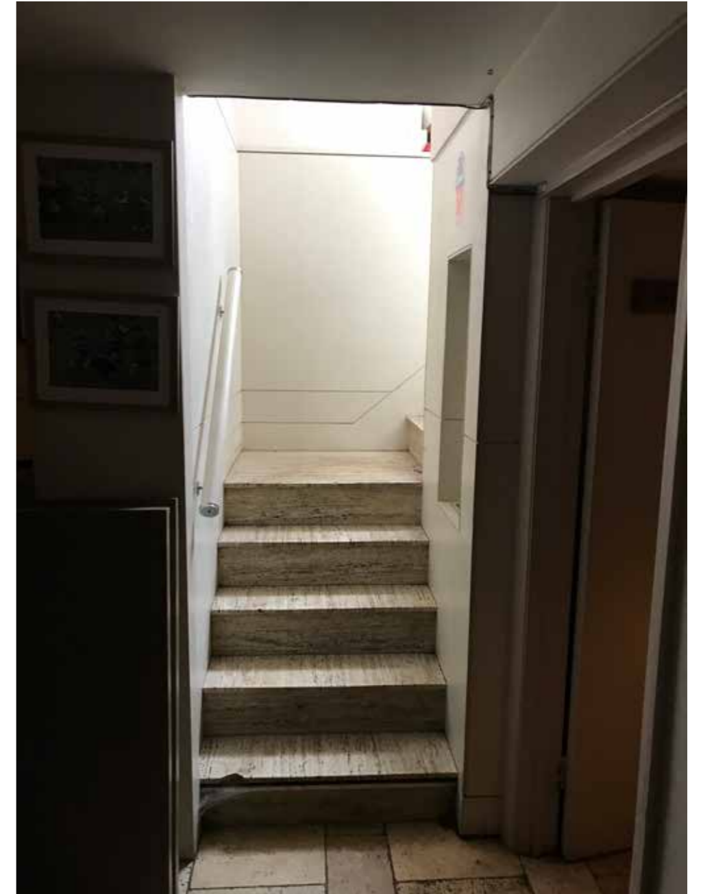
Stair from ground level to basement
