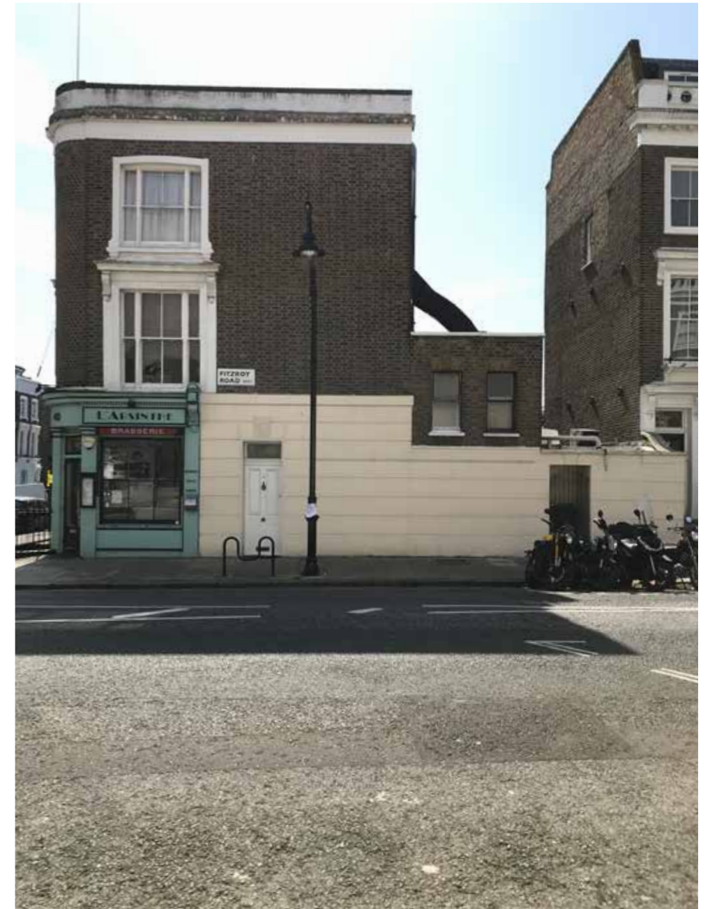
Existing frontage to Fitzroy Road
