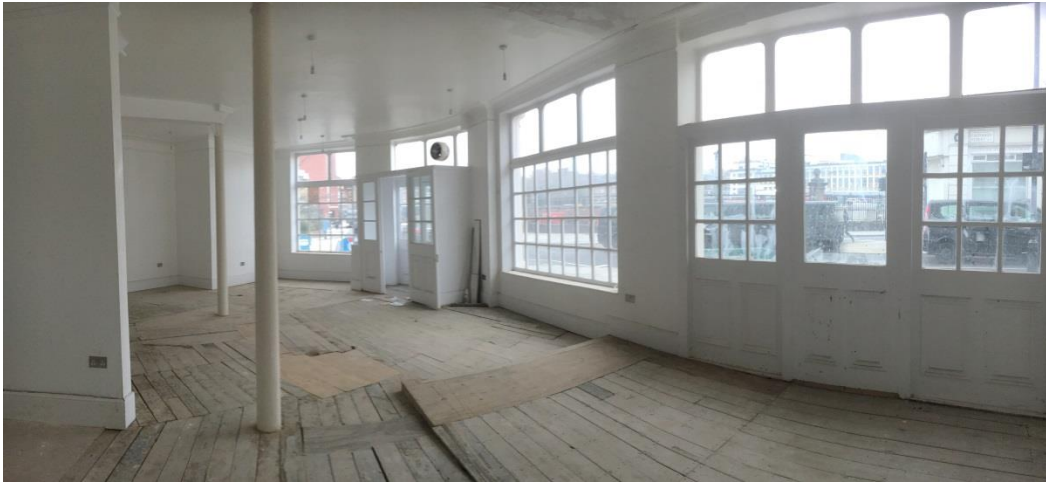
Figure 3.6 - The former pub premises at ground floor level.
