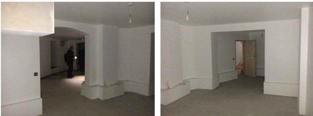
Figure 3.7 - The plain, utilitarian cellular spaces at basement level.
