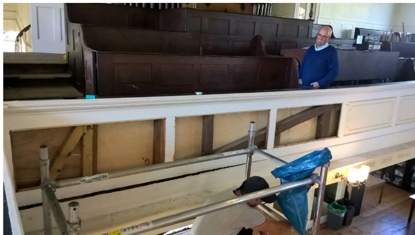
Photograph 13 Opening up to external face of balcony showing original truss members (dark) and new strengthening timbers (light)
