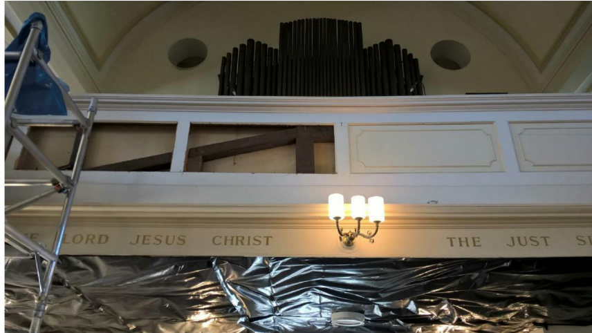
Photograph 12 Opening up to external face of balcony showing truss
