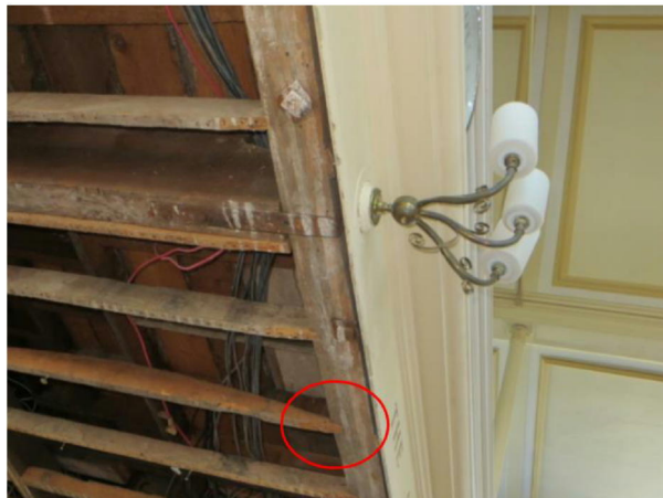
Photograph 6 Inadequate connectivity of ceiling joists
