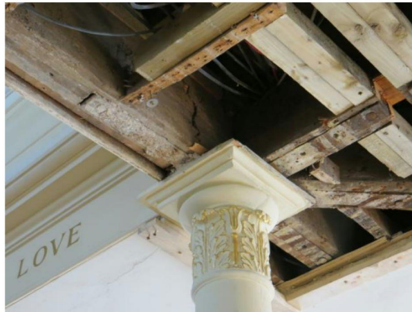
Photograph 10 Column head with incoming cracked edge beam
