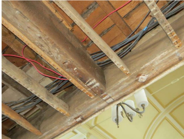
Photograph 11 Centre of transverse edge beam with incoming tie beam
