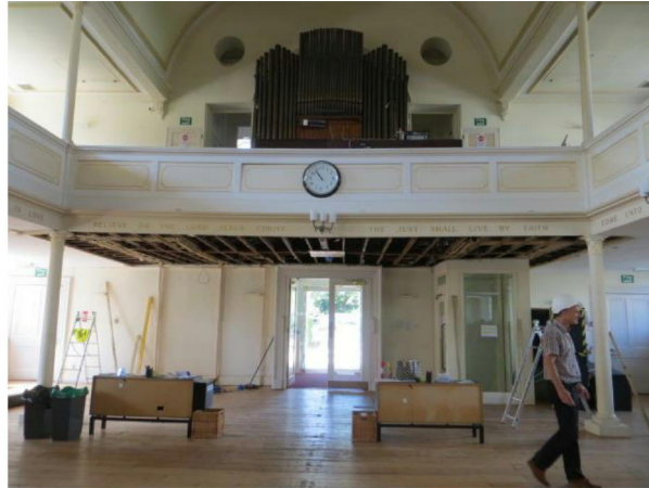
Photograph 1 General view of balcony, showing central deflection
