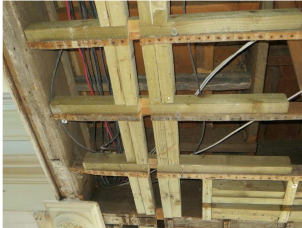
Photograph 5 Notching ceiling joists and strengthening
