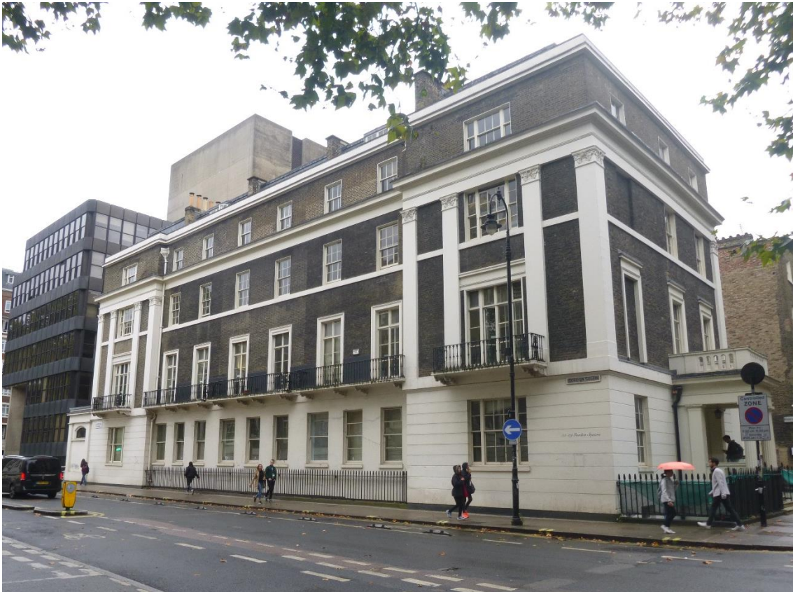
Fig. 8: Nos. 55–59 Gordon Square today, viewed from the north-west. The front doors of Nos. 56–58, in the centre, were converted into windows in the 1970s, when the road was extended over the front light wells
