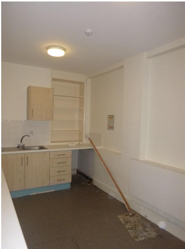
Fig. 19: Blocked windows in the front room of No. 56
