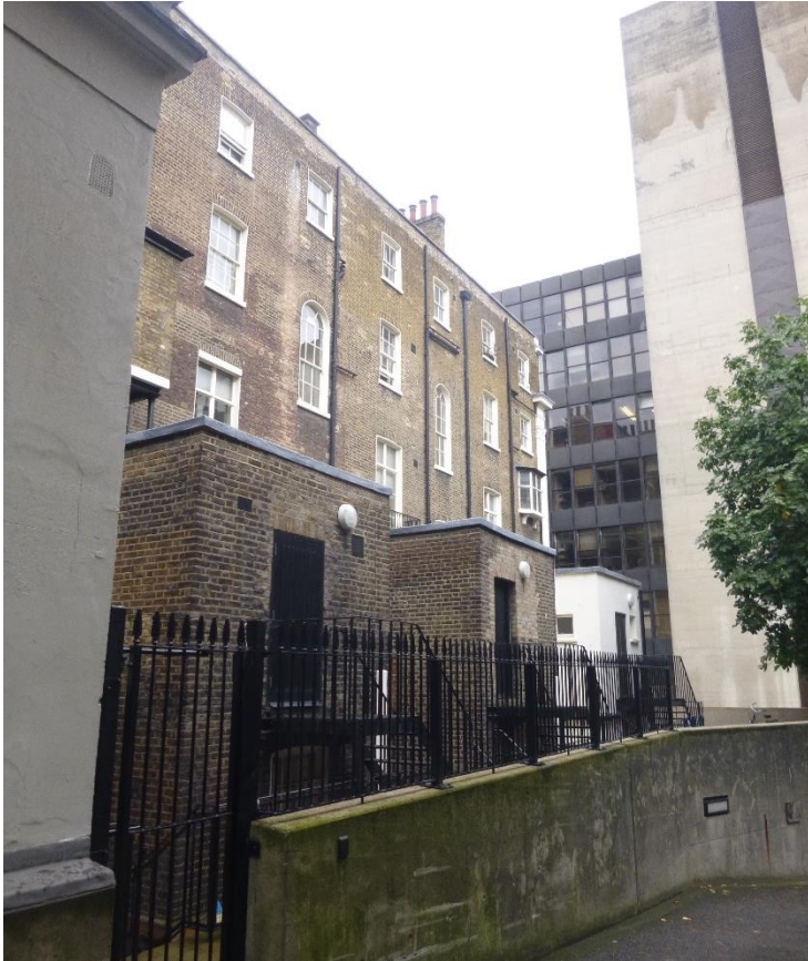
Fig. 11: Rear (south) elevation. The ground-floor window openings of the original closet wings of Nos. 56–58 have been converted into fire-escape doors
