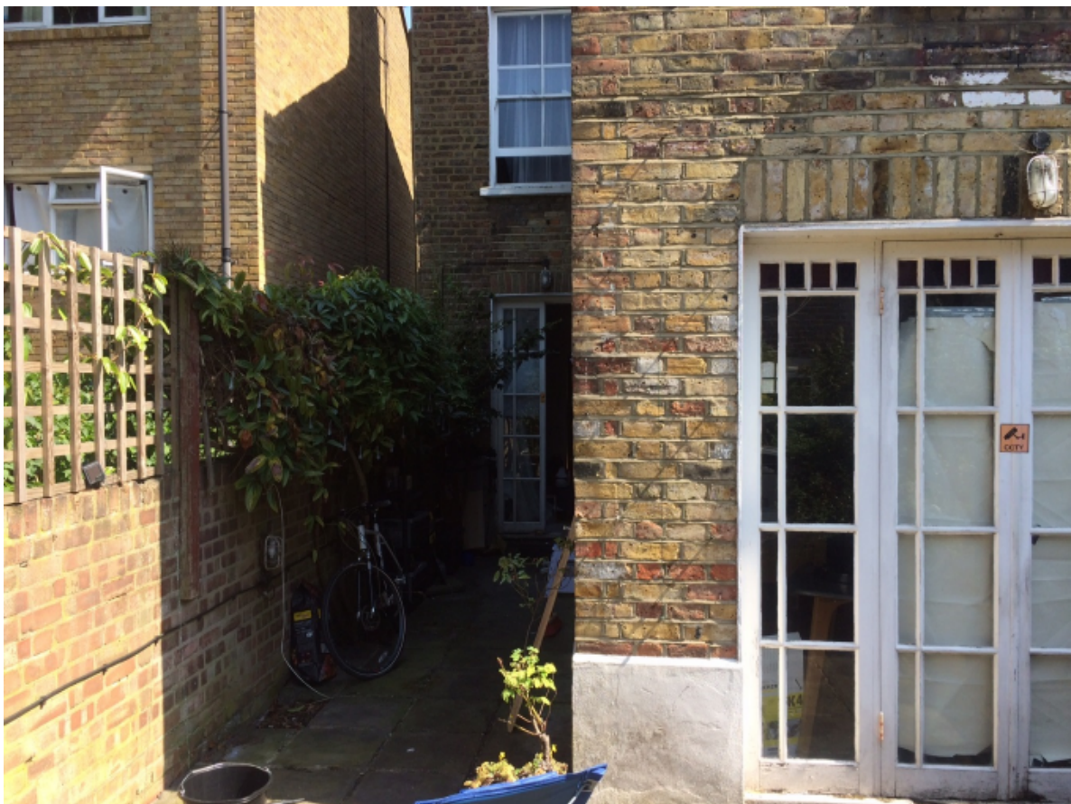
2. View of the existing gap to be infilled by the proposed extension, existing boundary wall and existing doors into the rear return at ground floor level – opening to be retained.
