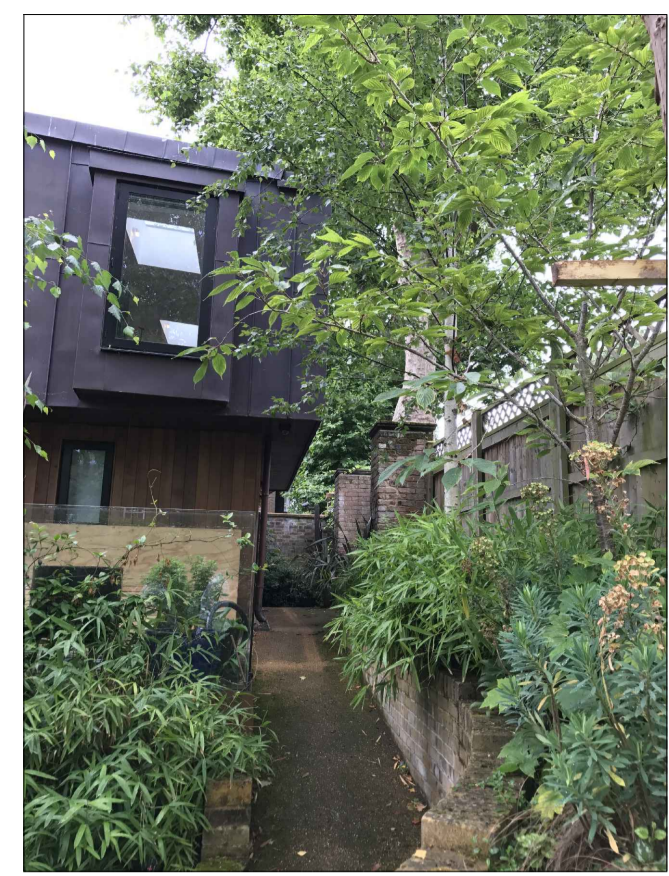
View from garden towards Tree house
