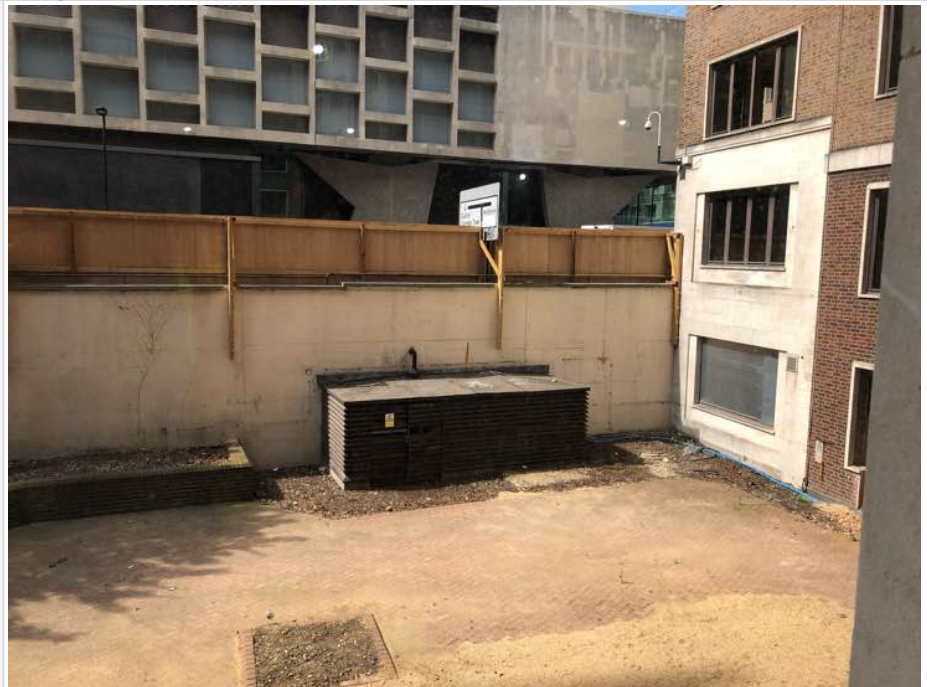
A further example of the perimeter where we will install metal perimeter bait stations
