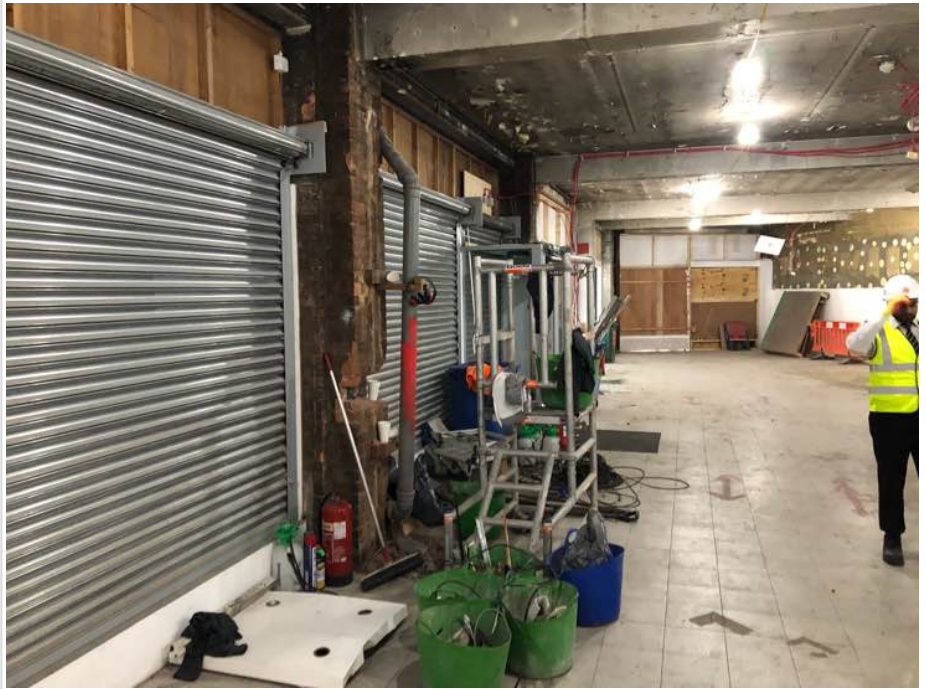
This picture shows the inside of Medius house we will install bait stations to the ground and basement level to control foraging rodents
