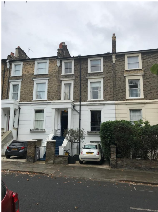
Fig 9 The front facade of the building.
