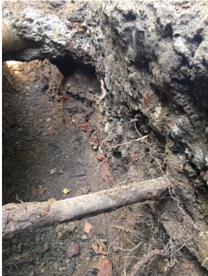
Profile of trial trench showing foundations to wall For this section beneath gas pipe some adventitious fibrous to 10mm root development
