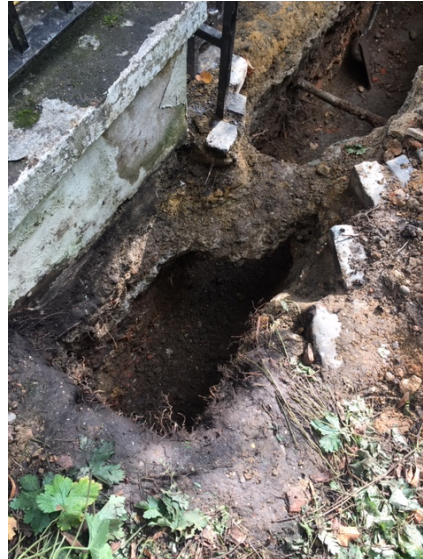
Build up of ground within trench showing wall base extending 200mm below ground level with and further 200mm foundations with significant made up ground beneath
