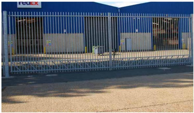
Barbican® swing gates are a perfect match to Barbican® fencing and shares all the principle design features of our fully welded pale-through-rail construction.
