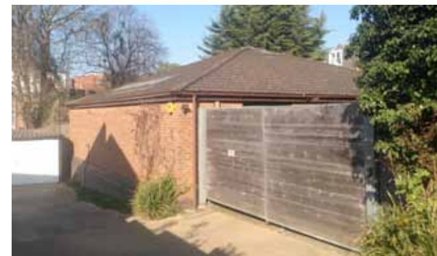
25 E Froggnal, a single storey house adjacent to the west of the site.
