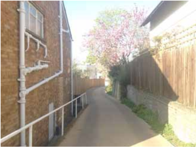
01 Entrance to private drive of 29/33 Arkwright Road accessed via Frogd.
