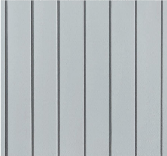
General view - showing vertical standing seams
