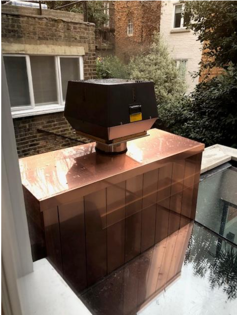
Photo 3 showing chimney from upper ground floor window
