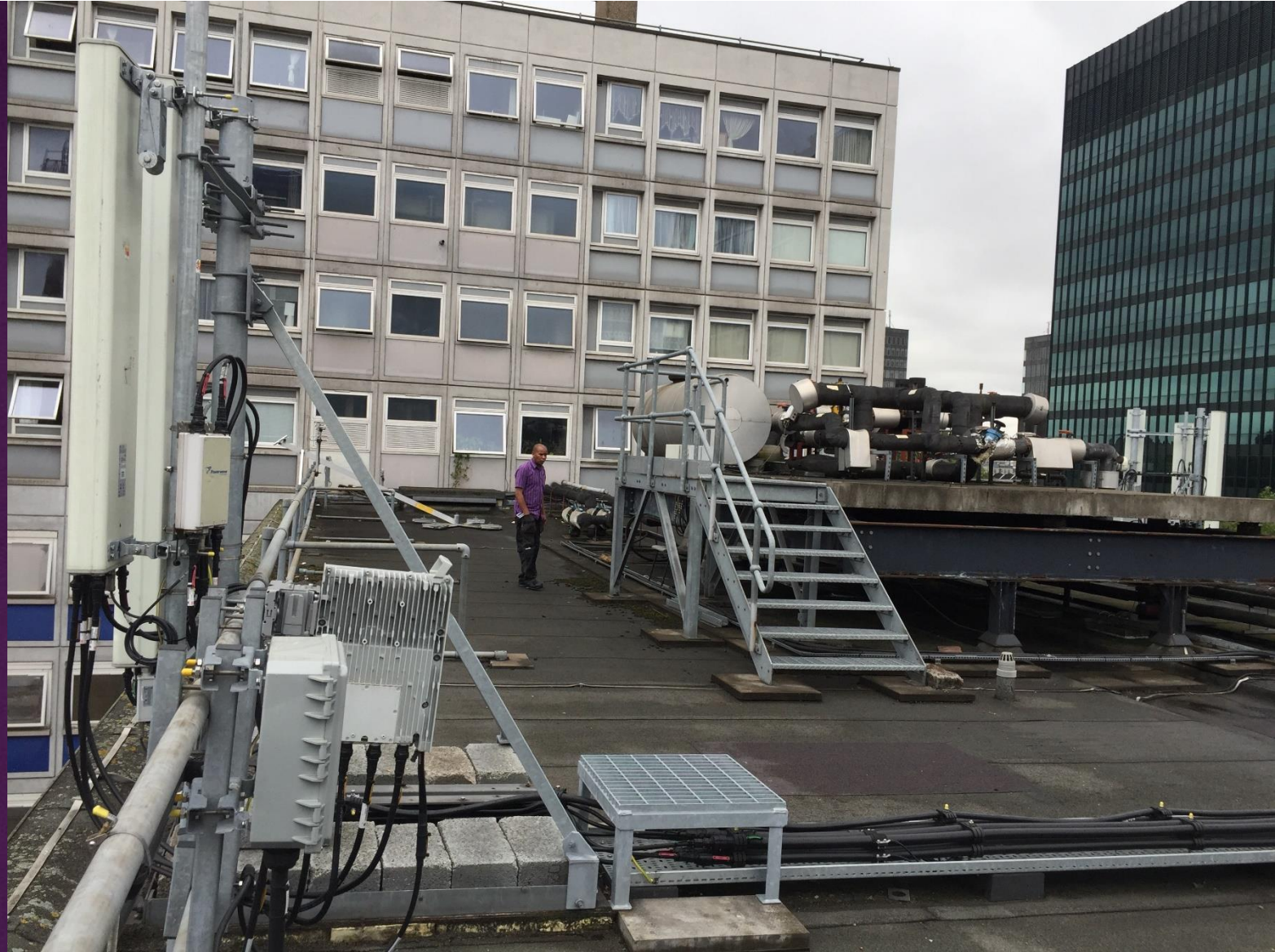
Roof Plant Area
