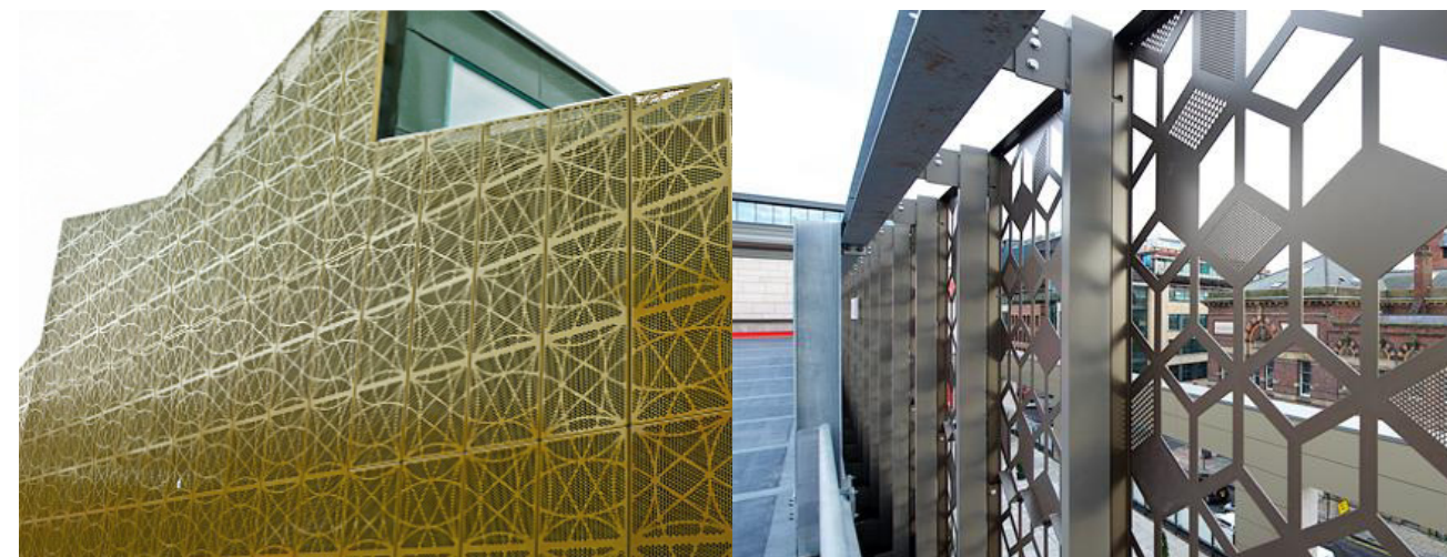
Feature Perforated Metal Cladding to Roof Extension
