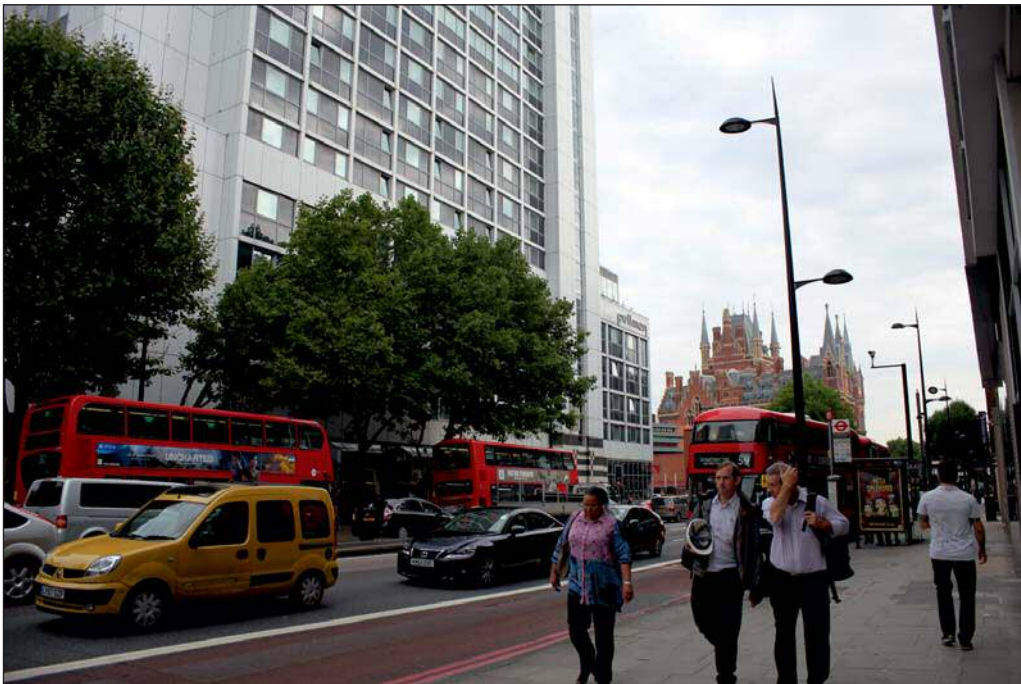
Plate 40: View from the Site looking north-east towards the Grade I listed British Library and St Pancras Station and Former Midland Grand Hotel. The latter lies within the Kings Cross Conservation Area
