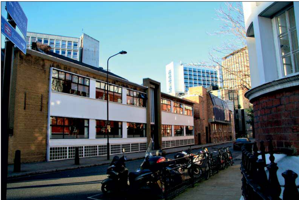
Plate 16: View from the south side of Flaxman Terrace at the junction with Burton Street, looking north towards the Site
