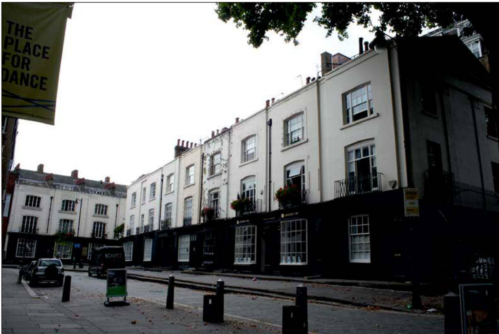
Plate 18: View of the Grade II* listed 2-16 Dukes Road (on the west side of the Duke's Road) and 4-18a Woburn Walk in the background. Both lie within the Bloomsbury Conservation Area
