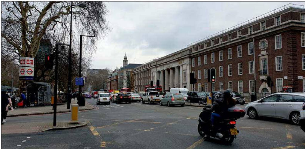
Plate 22: View looking east along Euston Road towards the Site from within Sub Area 1 of the Bloomsbury Conservation Area, showing the Grade II listed Drayton House Friends Meeting House
