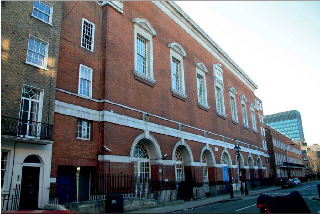
Plate 11: View of the rear of the British Medical Association building and 1950s extension at the northwest end of Burton Street
