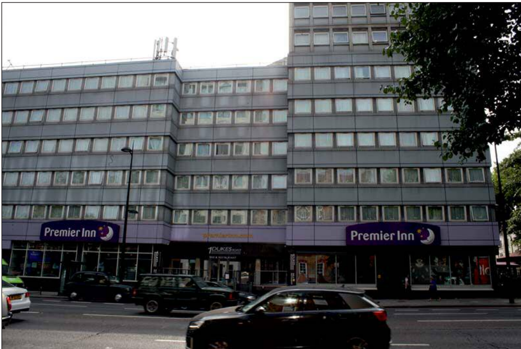
Plate 38: View of the Site from the Grade II listed Elizabeth Garrett Anderson Hospital
