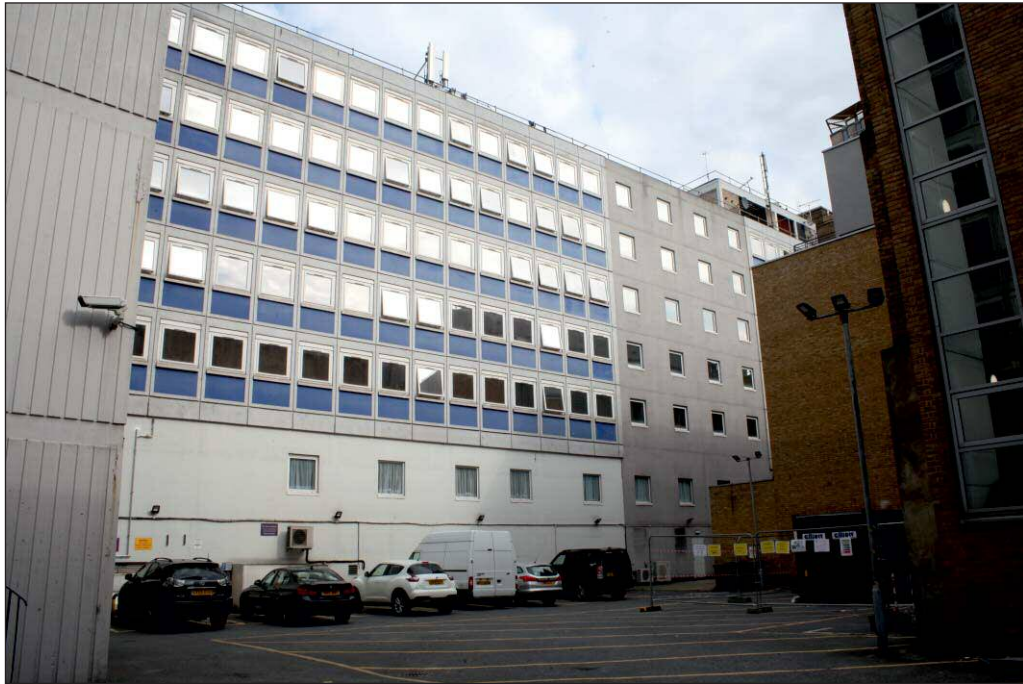
Plate 3: The rear of the Site viewed from the southwest showing the six-storey block and basement car park/service yard
