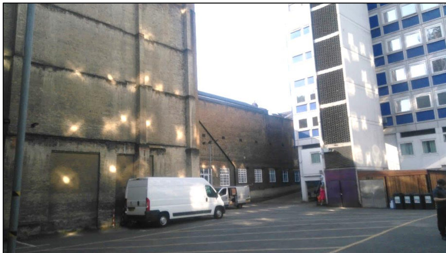
Photograph 6.1. On-Site Delivery and Servicing Yard
