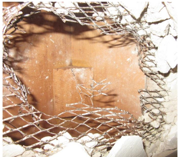
Figure 24: The structure of the 1950s staircase and its curved enclosure is made up of modern brickwork, metal laths and plaster.
