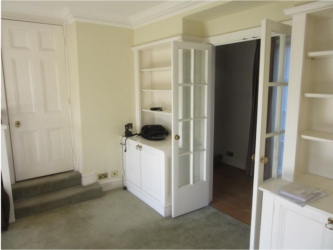
Figure 21: The 1950s configuration of the plan form partitioned the original front room to create an entrance hall; the doorway illustrates the change of levels to the carriageway extension; the joinery is all mid to late 20 th century.
