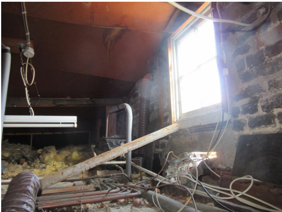
Figure 29: The roof structure within the carriageway extension appears to be 19 th century with mid-to late 20 th century alterations; the original valley gutter runs into the extension beneath the casement window.
