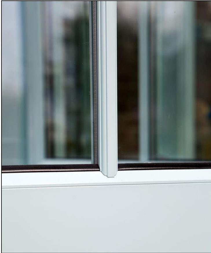
Proposed Narrow glazing bar, shown in light blue
