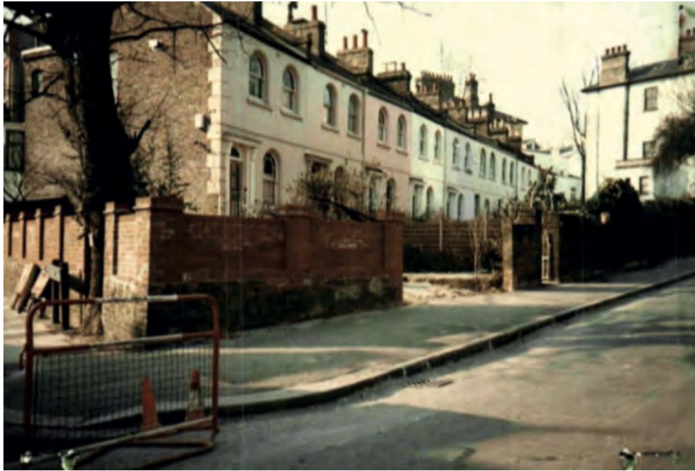
The boundary wall in 1986 during the formation of the vehicular gates. The wall post dates the 1930s inclusion of the side plot into the garden. Only the stump remains of the large sycamore tree that damaged the wall.
