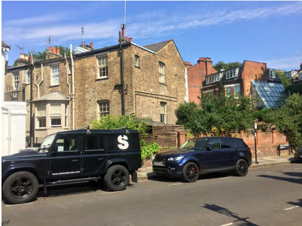
The rear and flank elevations of No 33. The flat-roofed, full-height rear addition dates from the early 20 th century (the bay to No 34 is later). None of the windows in the gable wall are original. A shed occupies some of the extension site. Note the variety of architectural forms and styles including the double height glazed extension on Willow Road opposite.
