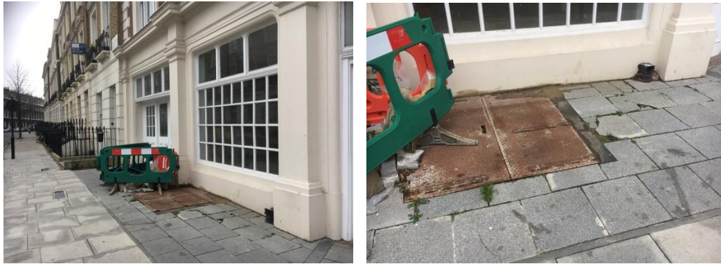
Figure 3.4: Functional / utilitarian barrel hatch set within the modern concrete paving around the former pub.
