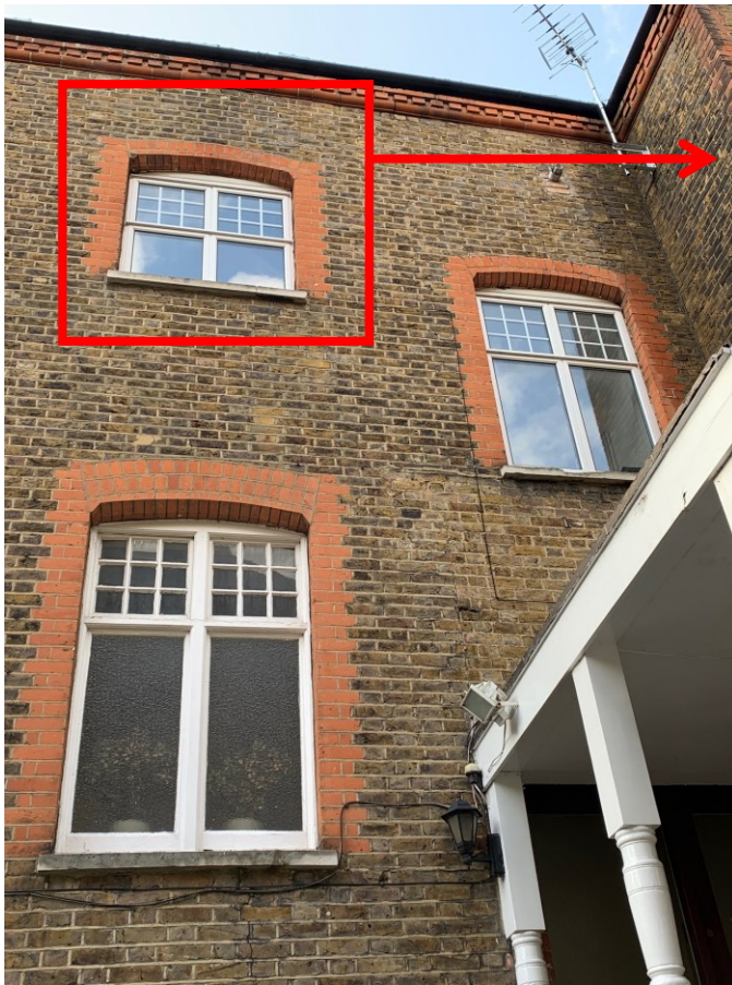
Close up of existing uPVC window with integrated glazing bars (Note: glazing bars are within the double glazing and not external to the window panes)
