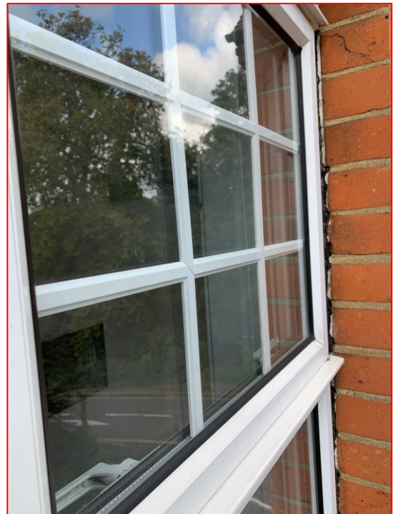
Close up of existing uPVC window with integrated glazing bars (Note: glazing bars are within the double glazing and not external to the window panes)
