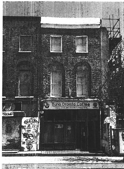
Pic 2 – View of front elevation
