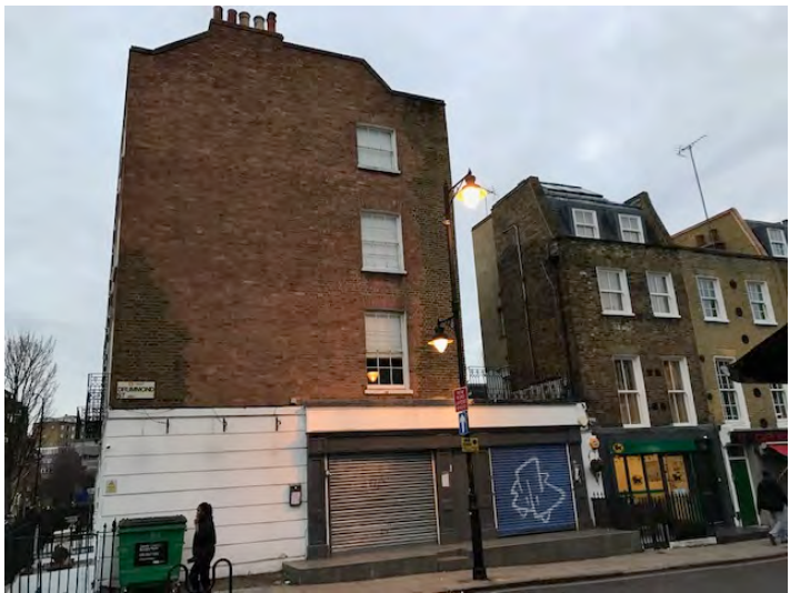
EXISTING PHOTO OF FRONT ELEVATION
