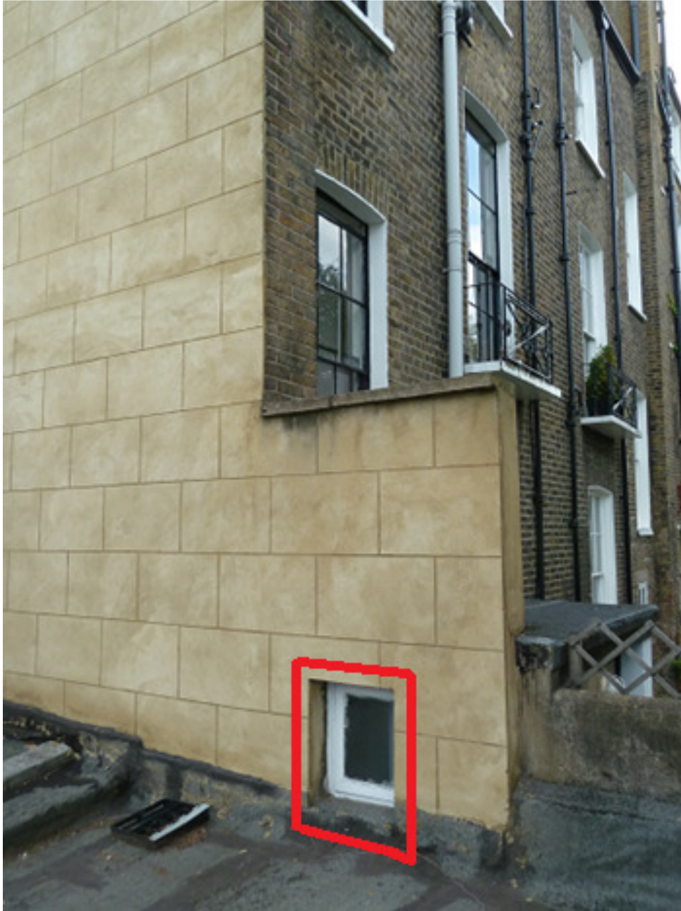
Photo 3: 24 Gloucester Crescent (side elevation)
