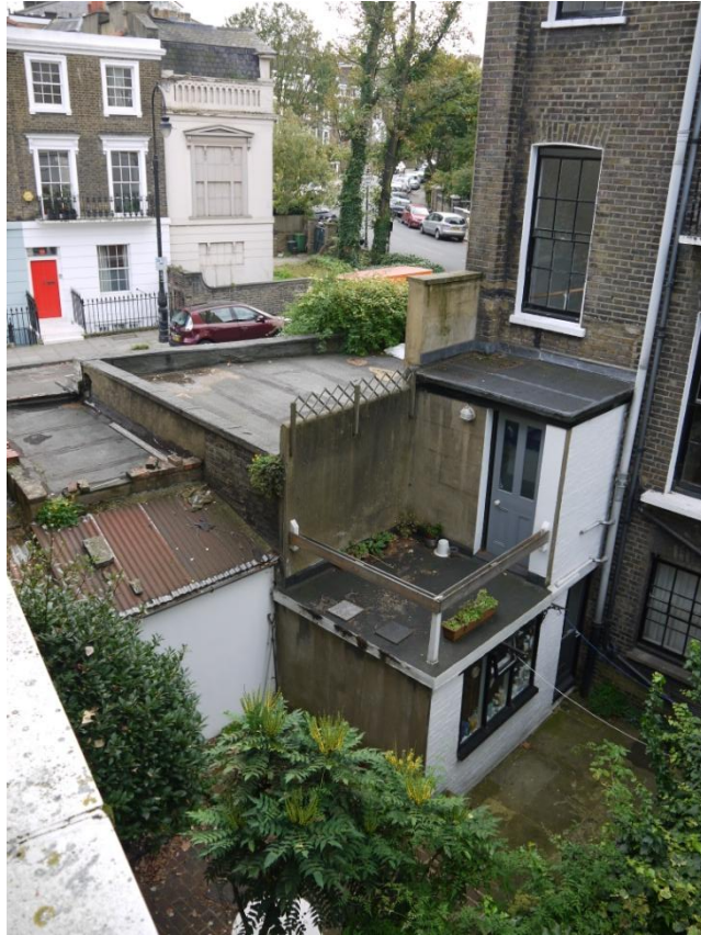
Photograph 3 - View from rear of No. 46
