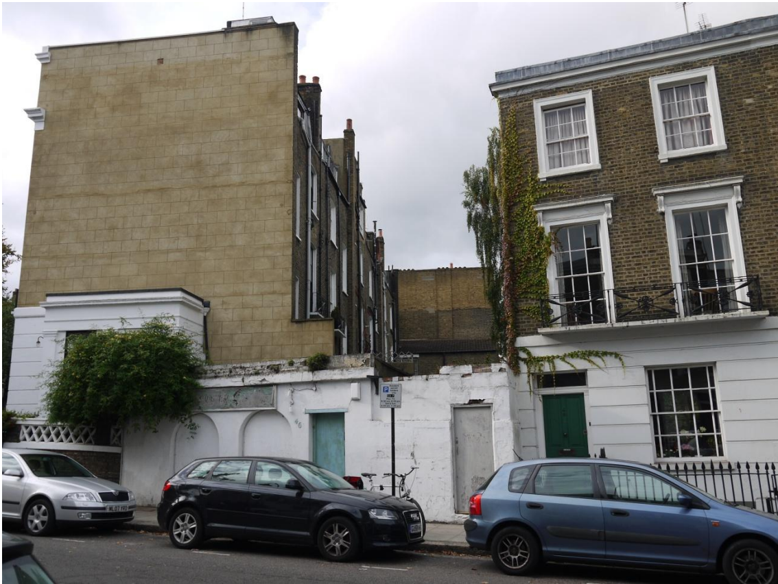
Photograph 1 - Front elevation of single-storey building at No. 46 Inverness St.
