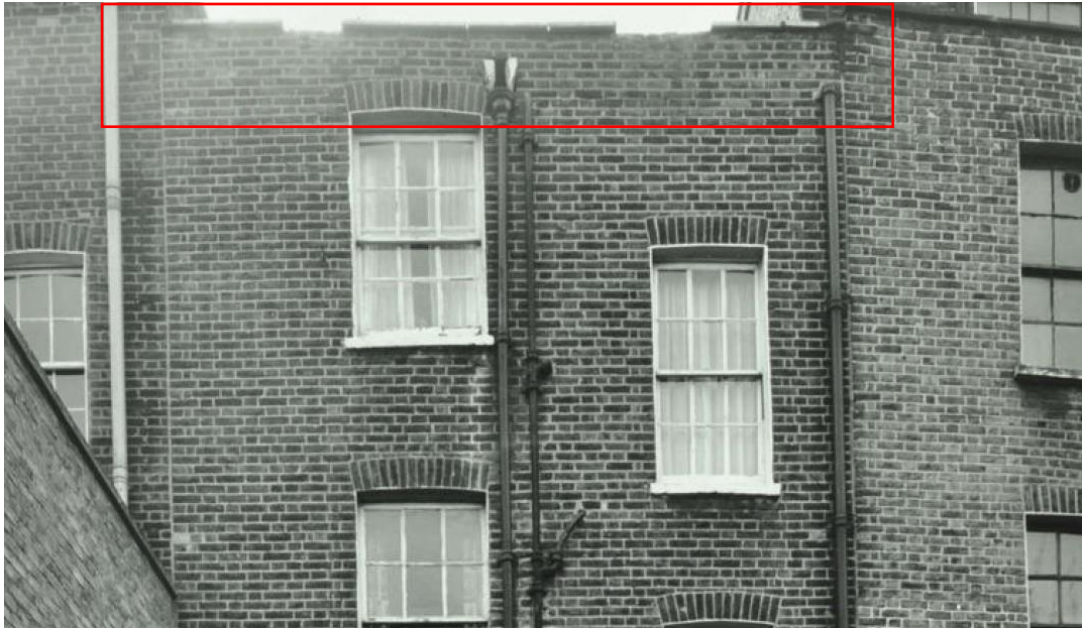
Fig. 5 Photograph. C1974 focused on roof area
