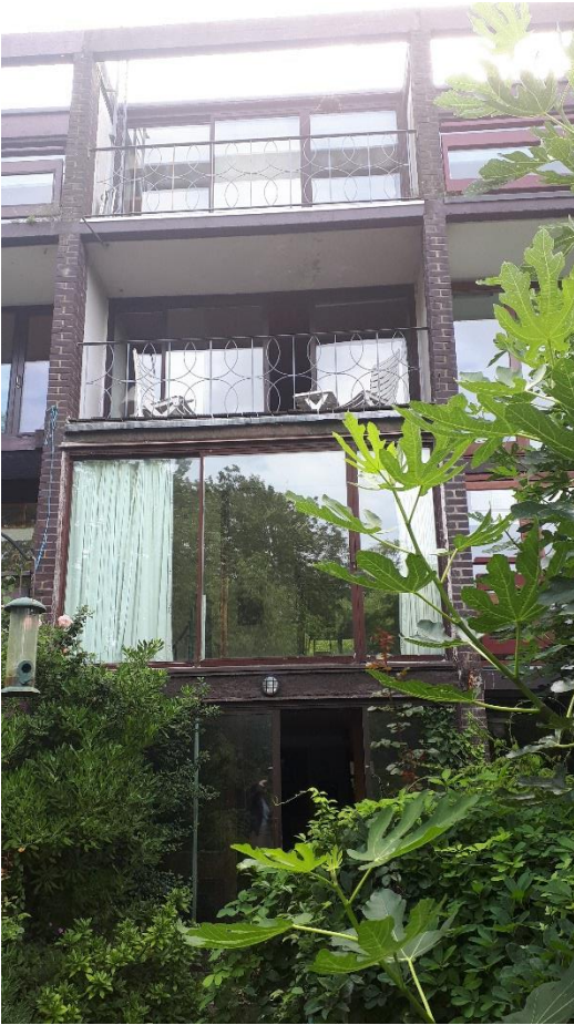
View of rear elevation
