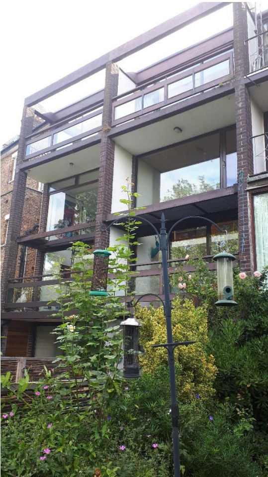
View of rear of No. 88
