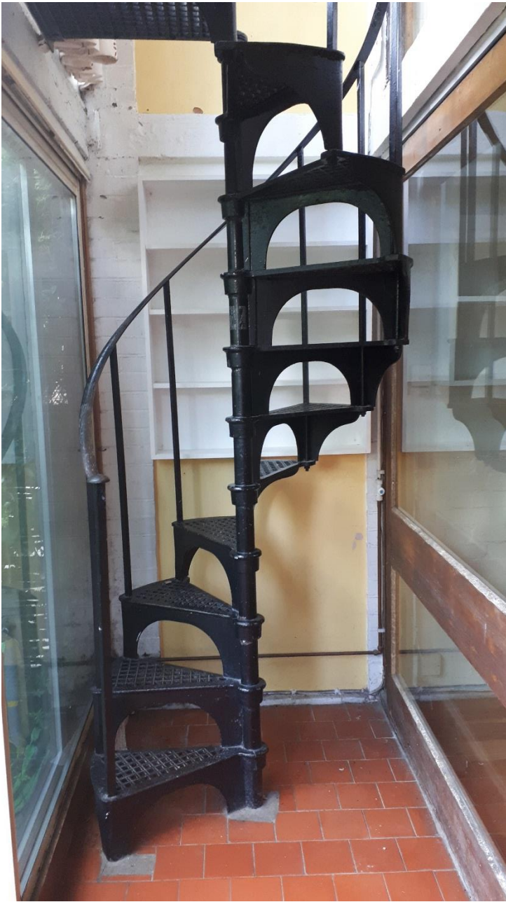
Existing spiral staircase on former open balcony, now enclosed
