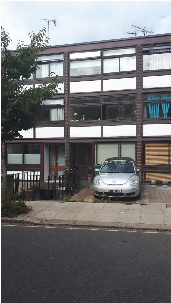
Front elevation of No. 86
