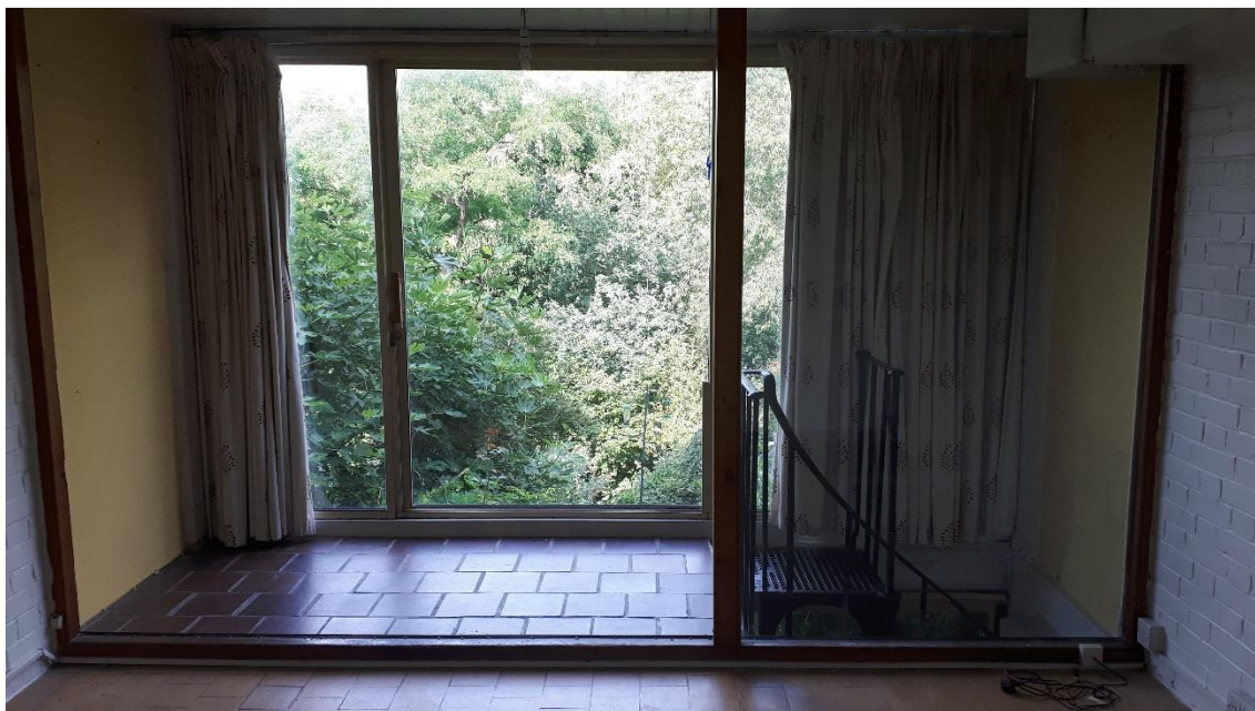
Upper ground floor – looking to rear from within the flat
