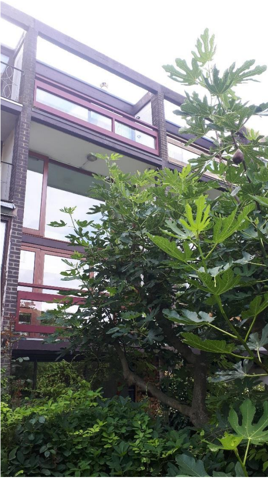
View of rear of No. 84
