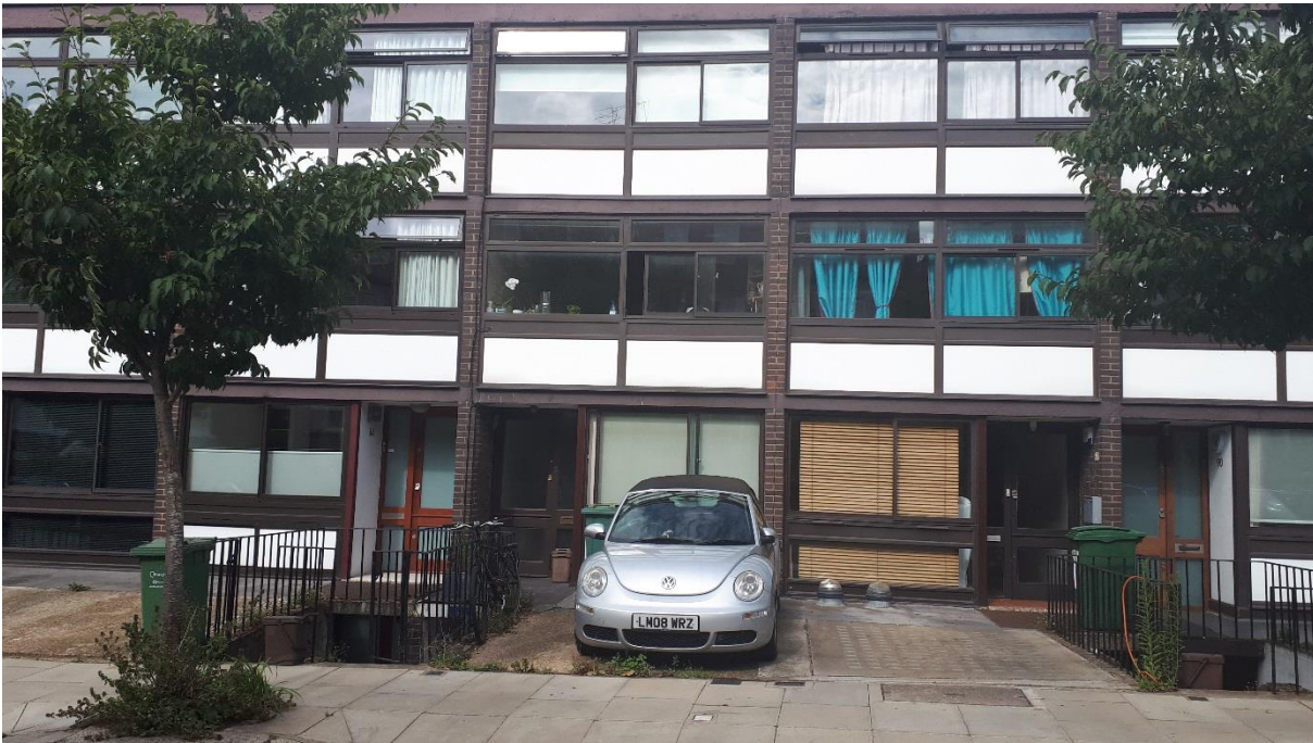
Front elevation of wider terrace
