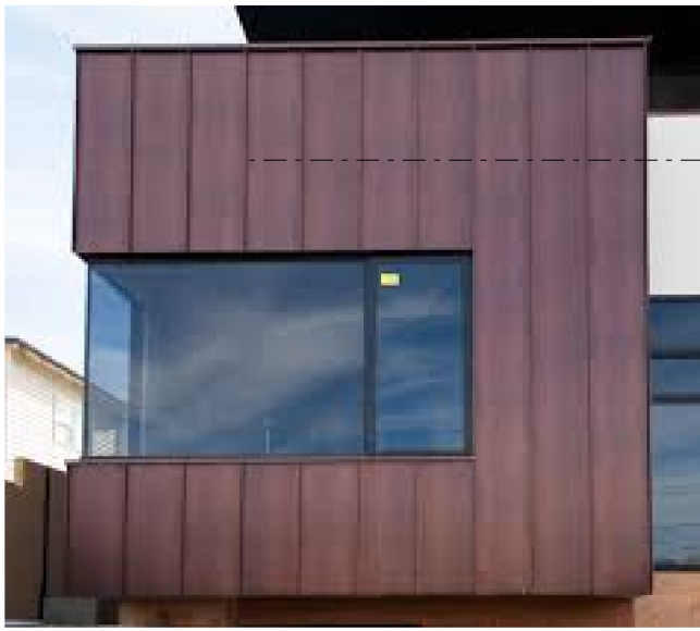
Key Ref No 2. Oxidised Copper vertical Standing Seam Cladding
