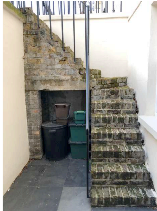
PHOTOGRAPH 02. VIEW OF MODERN BRICK STAIR FROM LIGHTWELL
