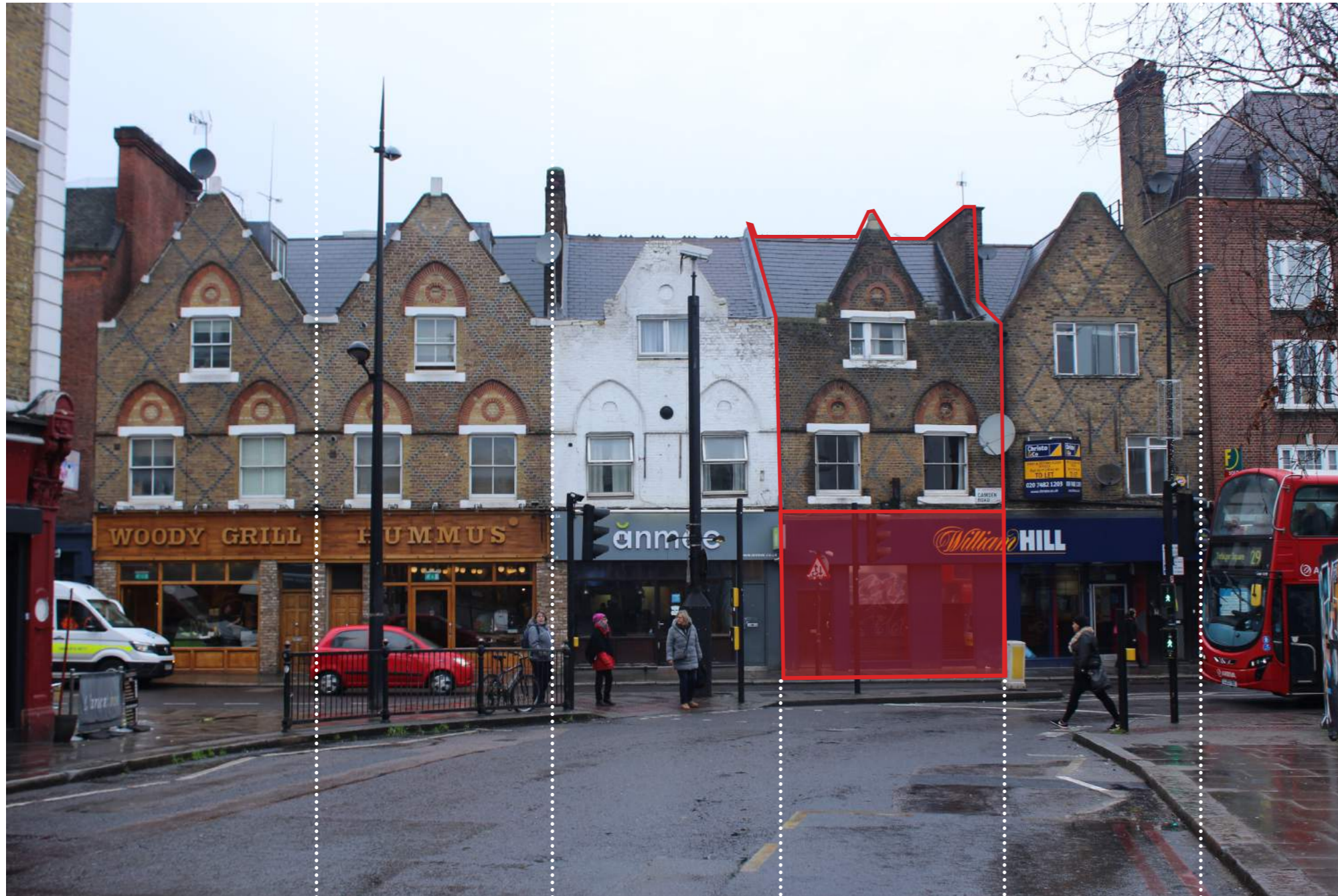
1a Camden Road
