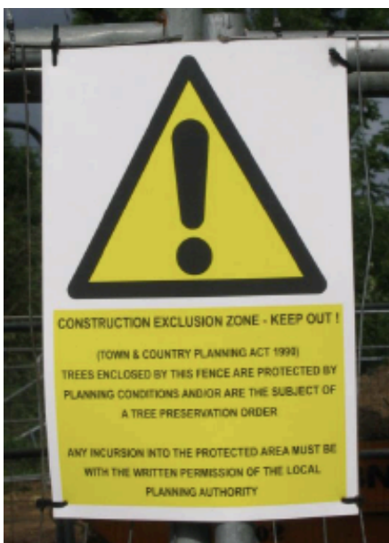
Figure 2 – Example of suitable warning sign affixed to protective barrier
