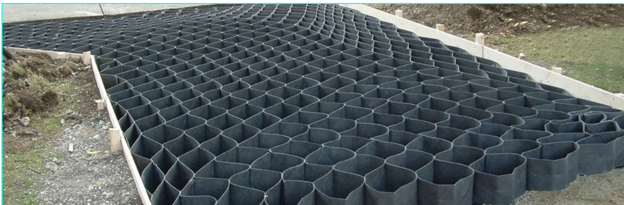
Example 3-d cellular confinement system prior to installation of stone.
