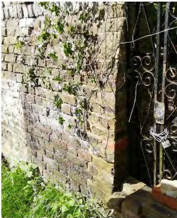
Photo 5, new/old brickwork at opening reveal
