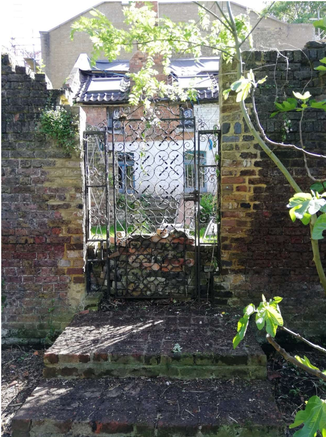
Photo 15, Opening 1 with new brickwork evident
