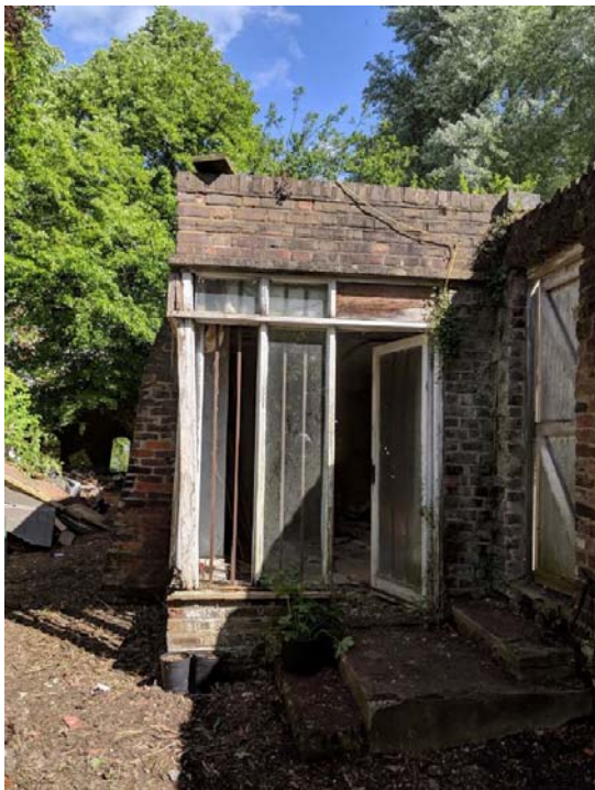
Photo 3: Outbuilding as viewed from No. 22 Frogmal Way
