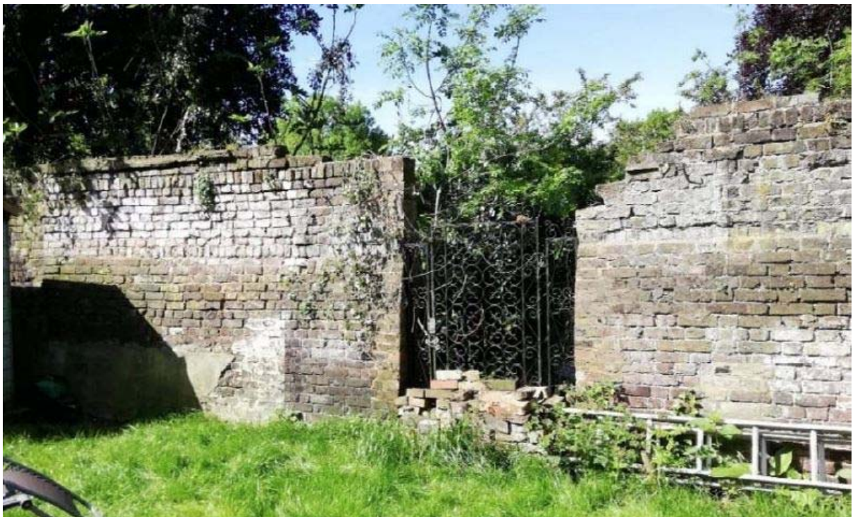
Photo 6: Boundary wall as viewed from No. 20 Perrin's Walk
