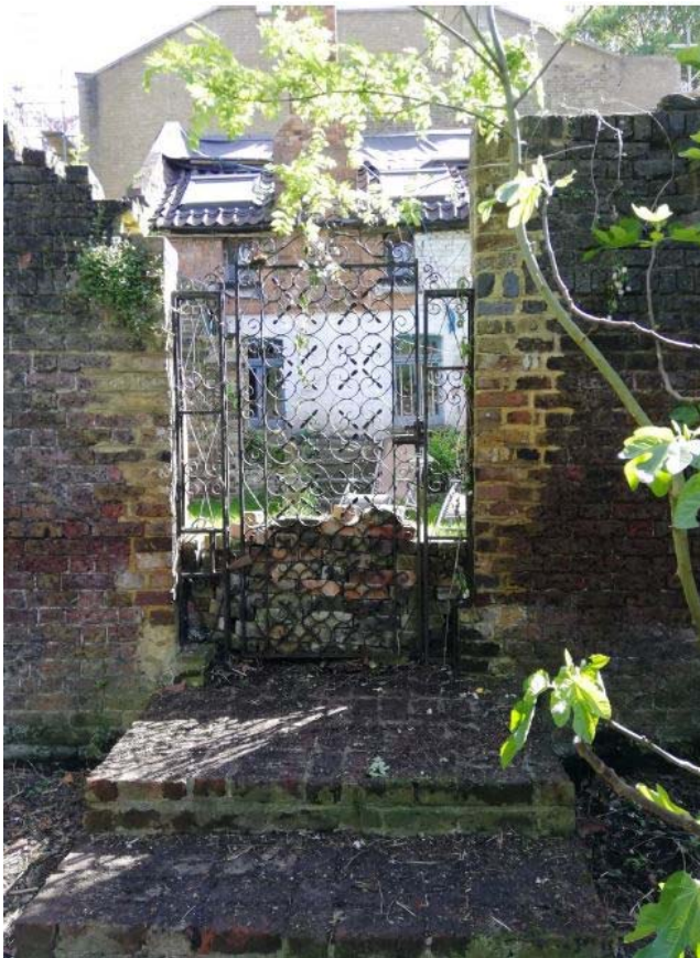
Photo 1: Metal gate – front view as viewed from No.22 Froggnal Way
