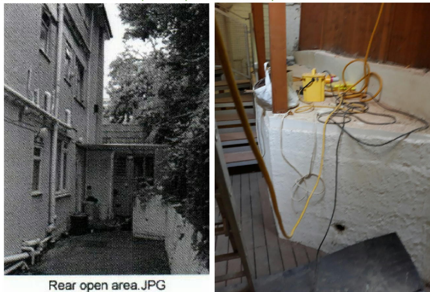
Photos above show an original photo from the 2004 application, clearly showing the boundary retaining wall. The second photo shows the reinforcement added in 2005 which I believe is responsible for holding T1 Lime in place.
