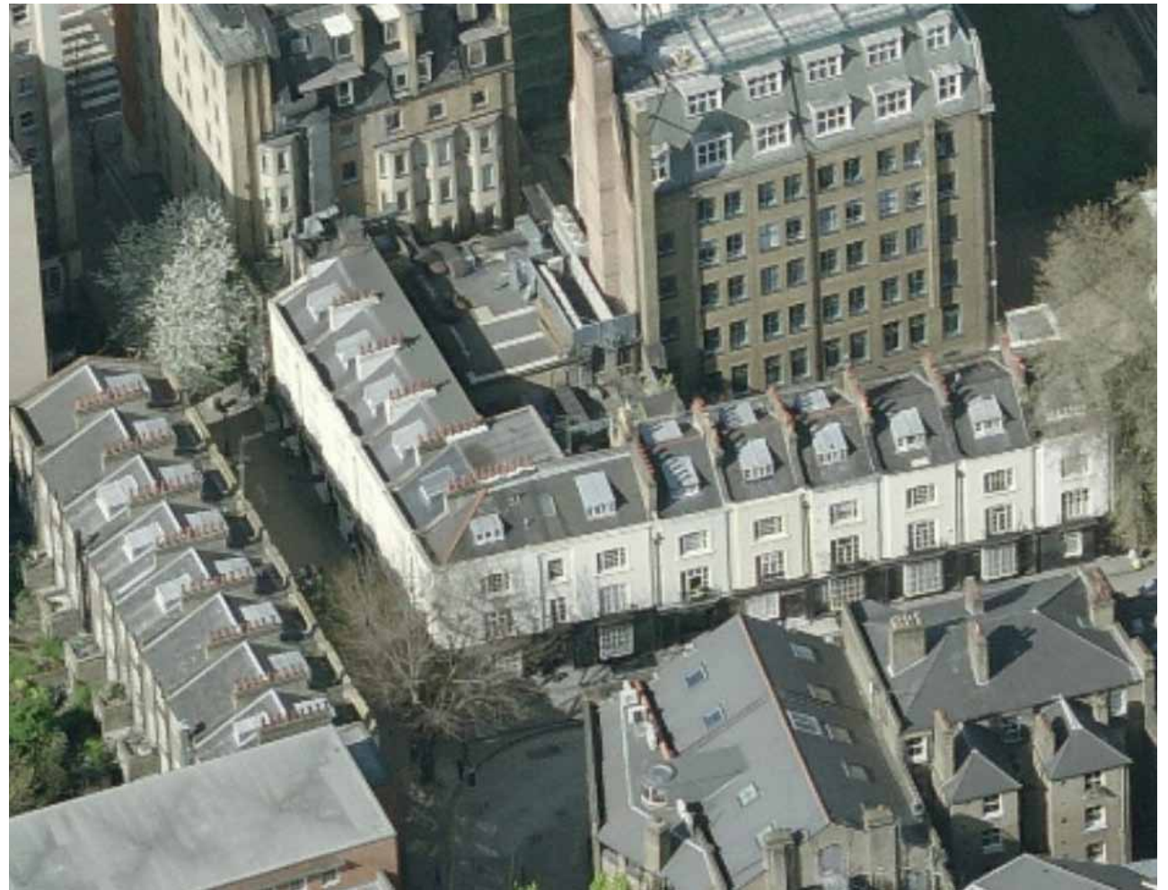
Aerial view looking West over the site.
