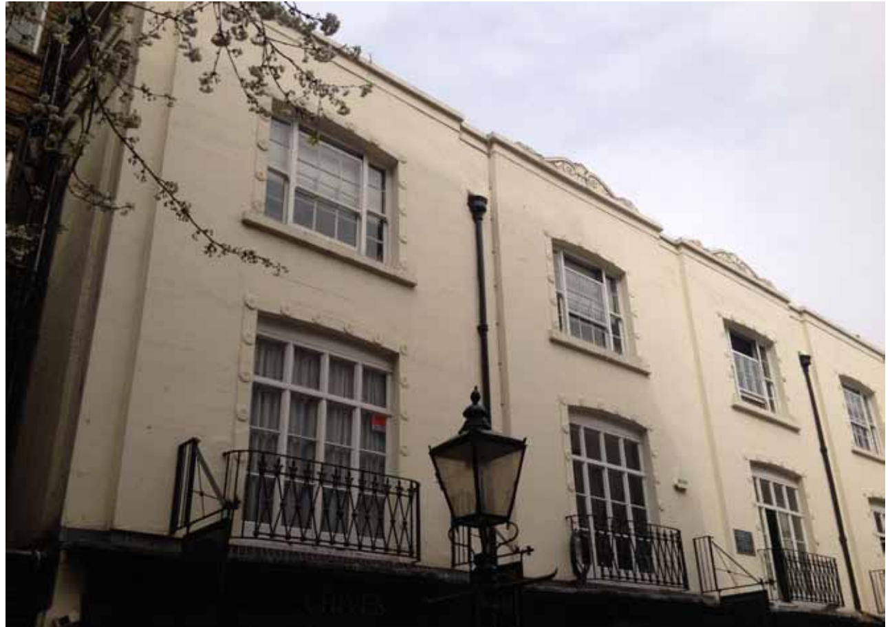
Front façade showing the first and second floor windows facing Woburn Walk. The plaque denotes the historic significance of its famous former resident.
