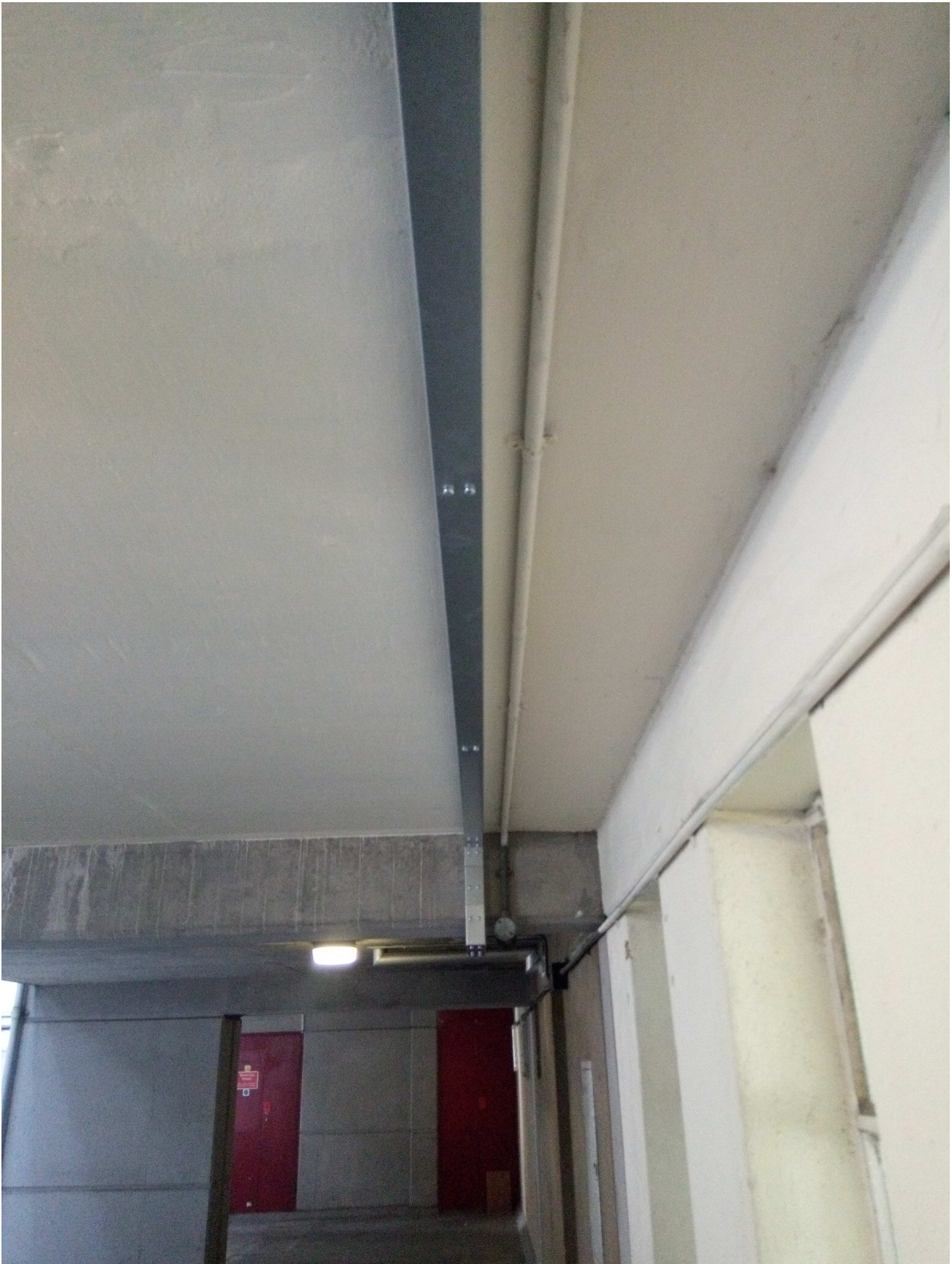
Sample square section trunking following route of existing retained tubular trunking outside 134 O'Donnell Court
