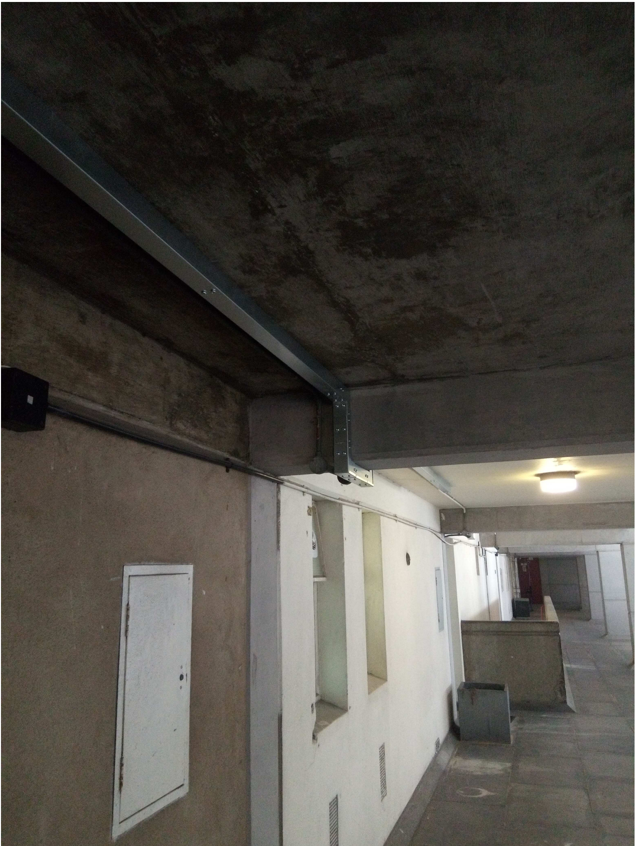
New trunking fixed in front of retained trunking
