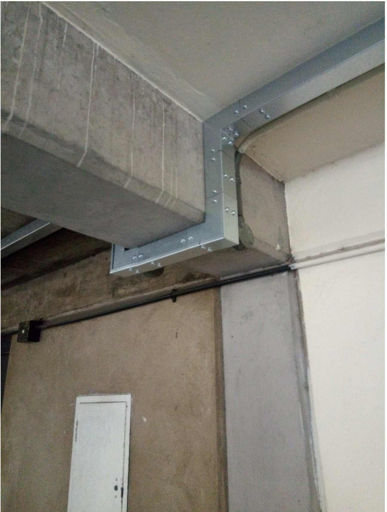
Detail at downstand beam, with junction box and retained trunking behind
