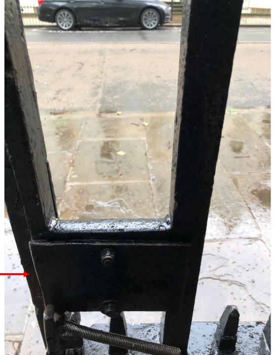
Cable Management to the lock will be via 10mm Steel tube which will be painted black finish and welded to the gate to run parallel with the cross beam
