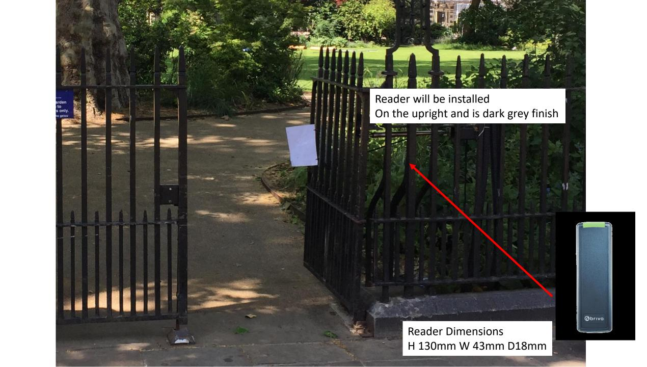
External Reader will be mounted on steel post which will be coated in Black finish RAL 9011 Graphite Black
