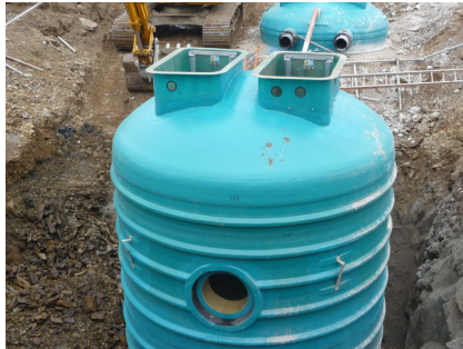
Large groutable inlet for concrete
