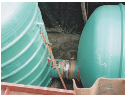
Flexseal coupling to connect all types of pipe up to 1200mm
