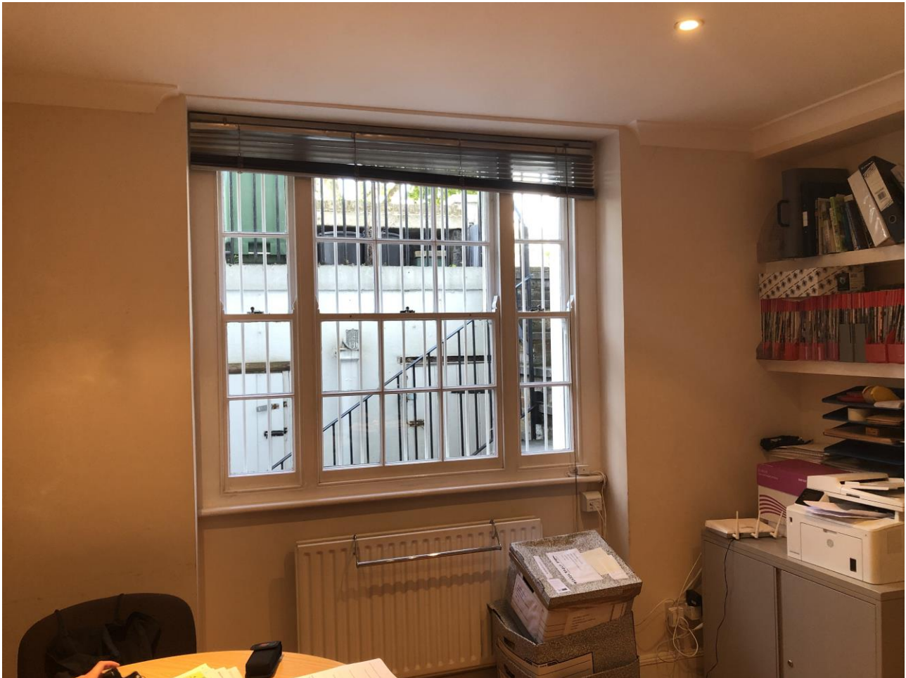
Figure 4: Internal view of the front external wall at basement level
