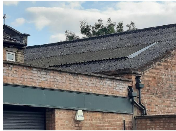
Plate 3.11 Asbestos Roof
