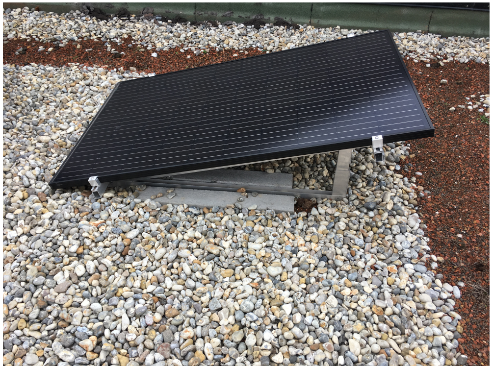
Fig 3 ballasted option which is closer to the roof substrate and therefore reduces the extent of green roof significantly
