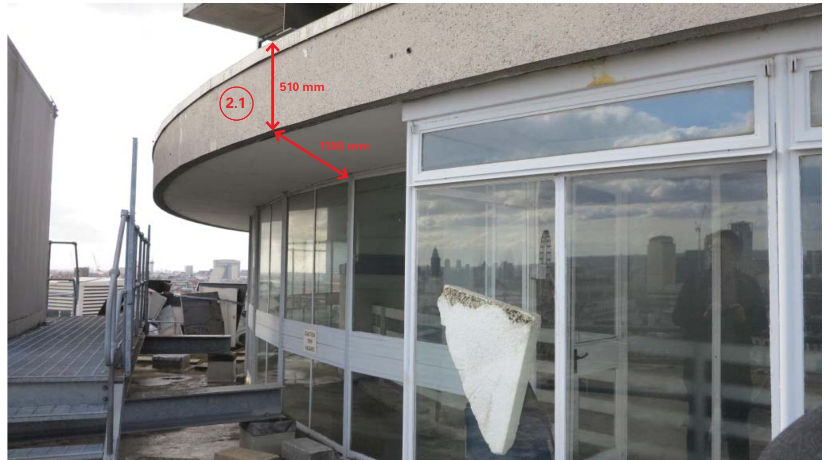
Dimensions of Existing Roof Overhang
