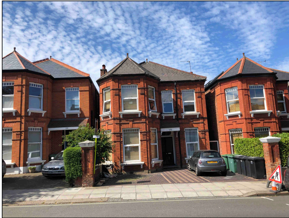
Figure 1: Photograph of the front elevation of the appeal property
