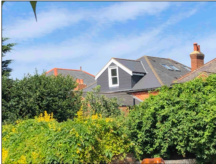
Figure 7: Photograph of a similar dormer on a property facing Manstone Road, and visible to passers-by from Fordwych Road
