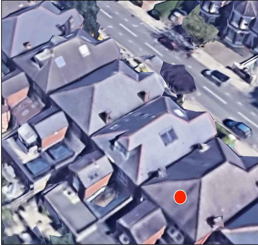
Figure 4: Satellite image of the appeal property (red dot) and dormers at numbers 128 and 132
