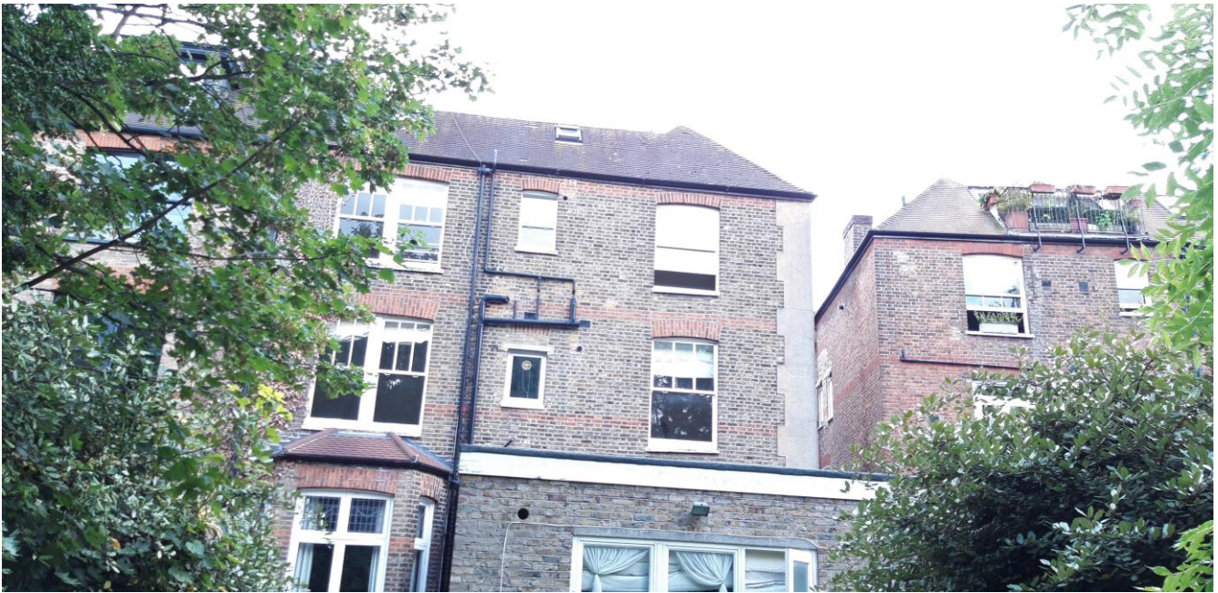
Photo 2 – Rear elevation showing adjacent dormer / balcony (No. 48 Canfield)
