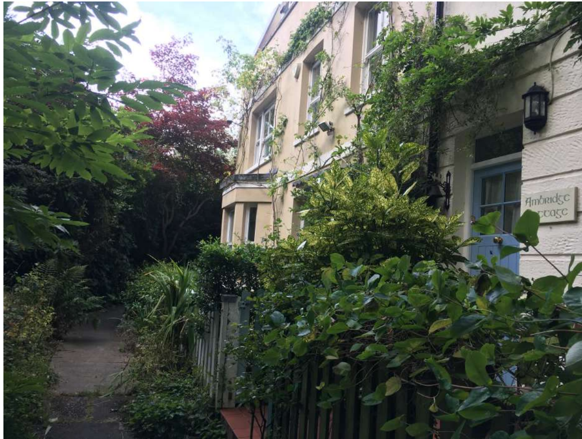
FRONT WITH THE EXISTING BAY
