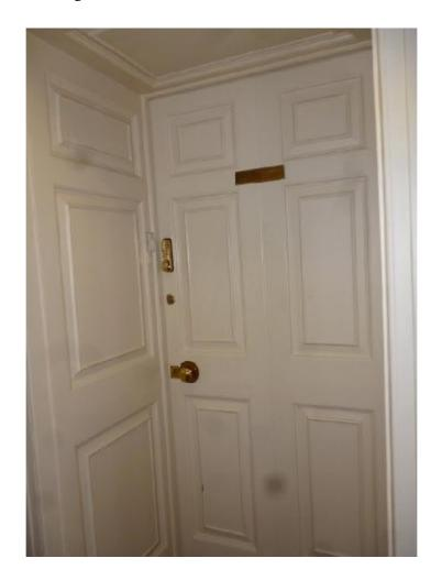
(ix) Flush panelled doors with staff bead panel moulds as on the illustrated existing oak and inner entrance door to the South Chambers
