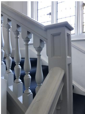
Figure 2. Main staircase at 39 Eton Avenue
