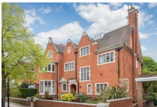
Figure 1: No. 39 Eton Avenue
